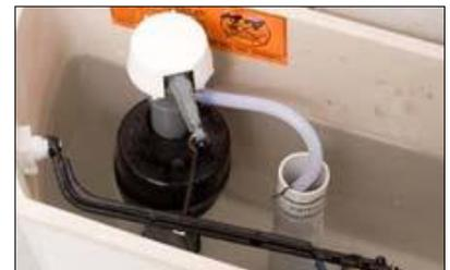
To detect silent leaks, remove the lid from the toilet tank, remove any colored or bleaching cleaning agents. Flush to clear the water in the bowl. Then add dye tablets, leak detector fluid, a few drops of food coloring, or a colored instant drink mix to the toilet tank. If there is a leak in the toilet, color will appear in the bowl within 60 minutes. Flush the remaining color from the tank as soon as the test is complete.
