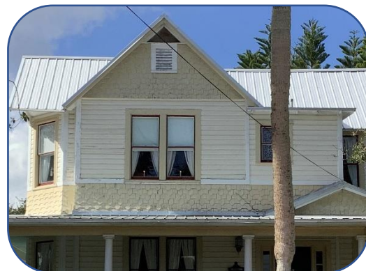
Figure 2: This well-preserved dwelling at 602 Indian River Avenue retains significant historic features such as original windows, wood siding, and decorative wood shingles that should be restored rather than replaced.
