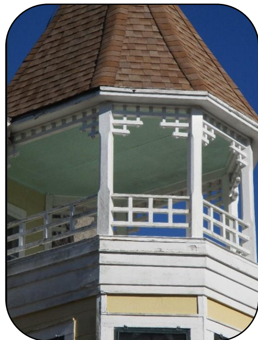
Figure 1: The wood trim on this balcony displays peeling paint and some damaged wood. Architectural features should be preserved rather than replaced.
