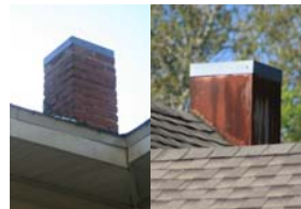
Brick and metal chimneys protruding from roof
