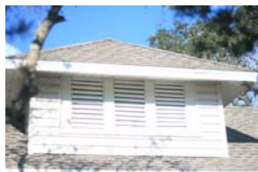
Dormer with battered vent casings
