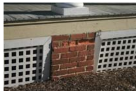
Brick foundation with lattice covering crawl space
