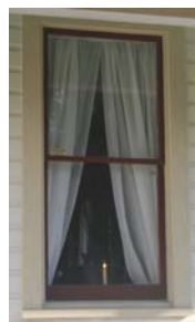
Original 1/1 double-hung sash windows
