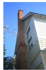
Chimney (west façade) with corbelled brick work
