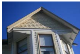
Decorative brackets above bay window
